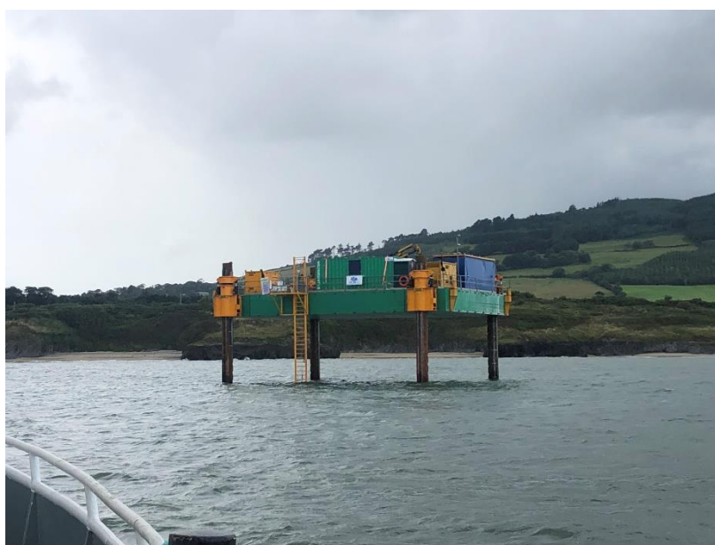
Figure 2-1: Jack-up Barge OCM 80
